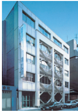
* Seismic Strengthening System with Supplemental Exterior Frame
