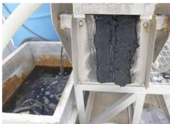
図 - 15 Dewatering of Scum by Screw Press
